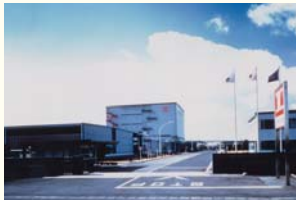
Komaki Plant (Certified under ISO 14001 in March 1998)
