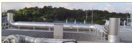
Spray-type odor elimination duct
