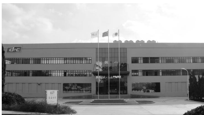
Production facilities for LC materials (PRC)
